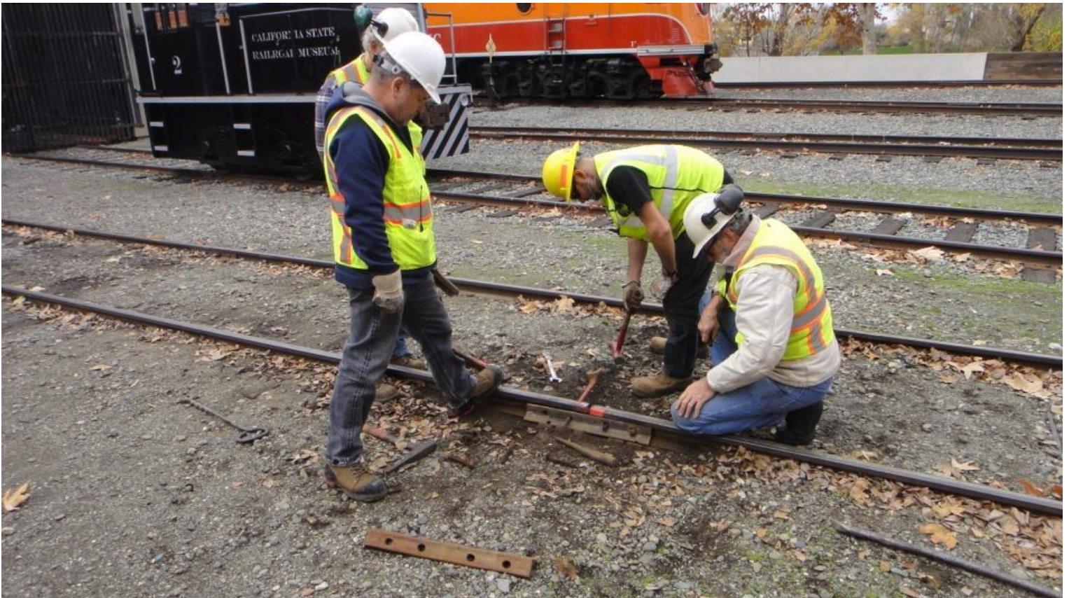
Chris pounds a drift-pin through the bolt-hole
