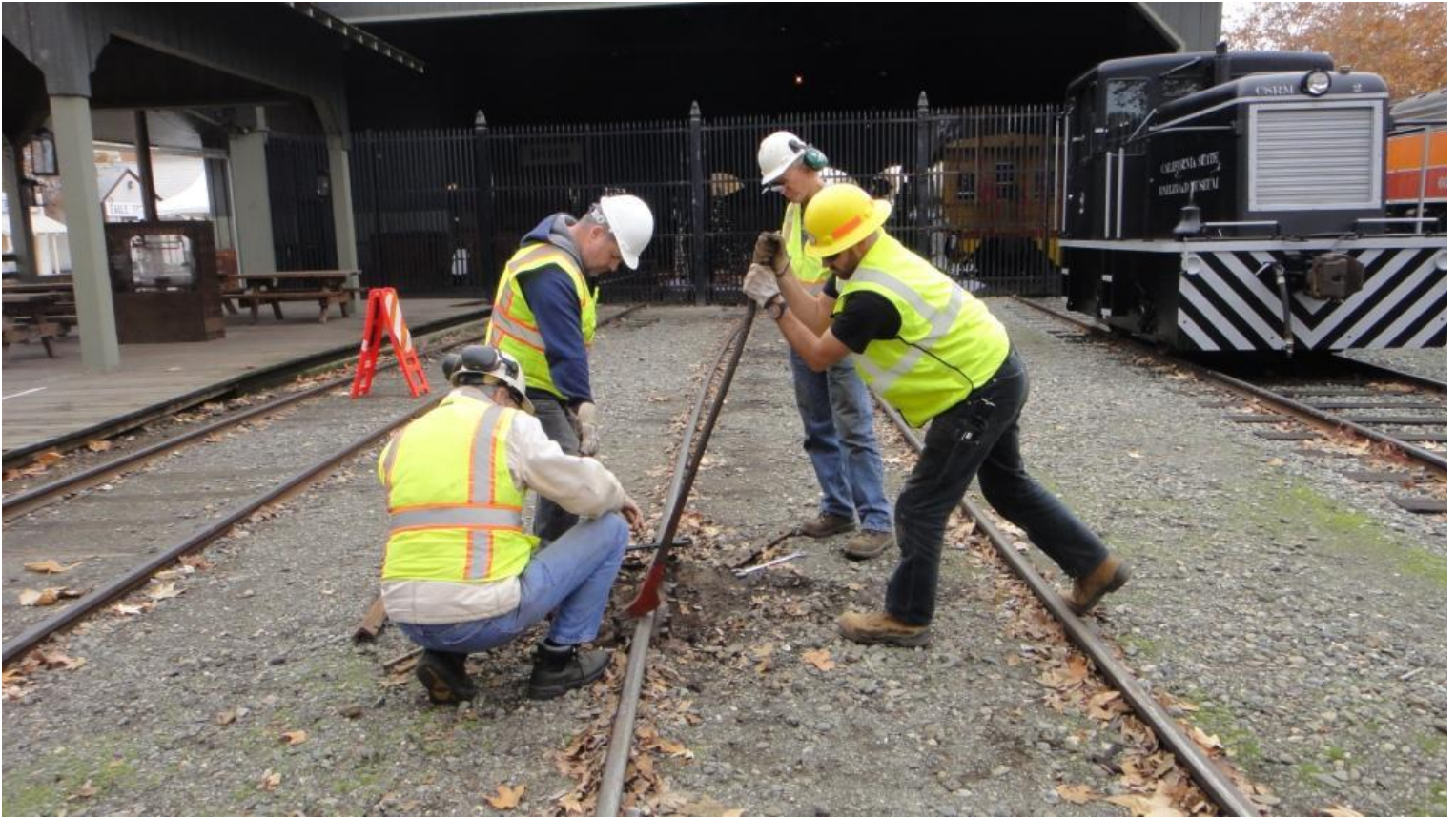
Steve W. holds the road-master on the spike-head while Chris uses the claw-bar to pull it
