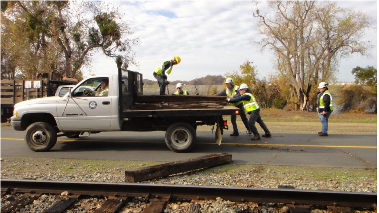
Alan drives the flatbed down the bike path stopping at each dead tie as Steve N. and Steve W. lift the ties which Chris pulls aboard
