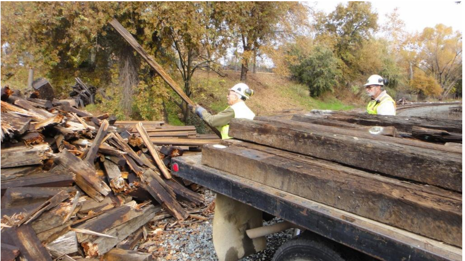
At Setzer, Clem tosses a piece of tie onto the pile
