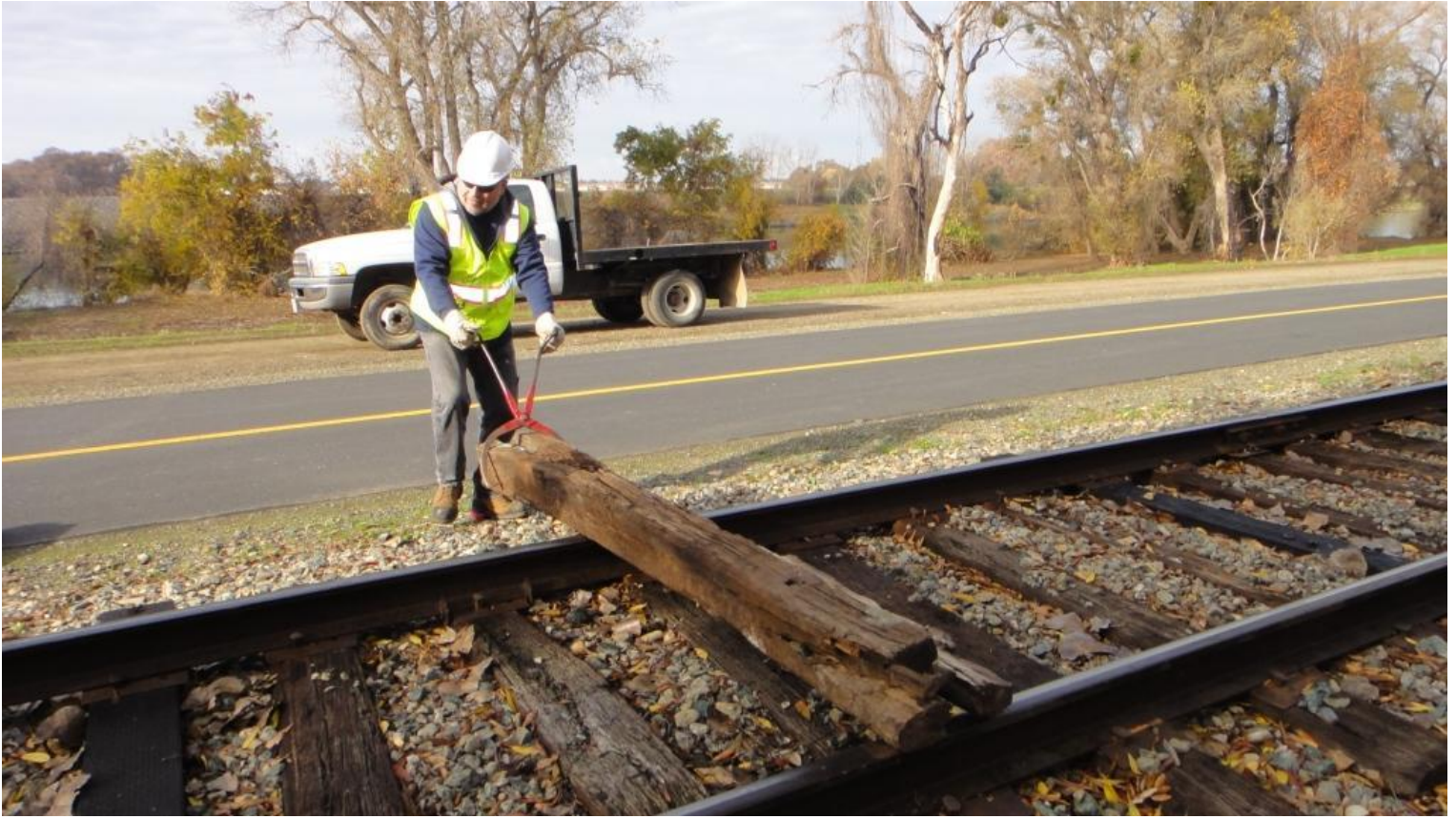
Steve N. pulls a dead tie on to the rails staging it for pick-up
