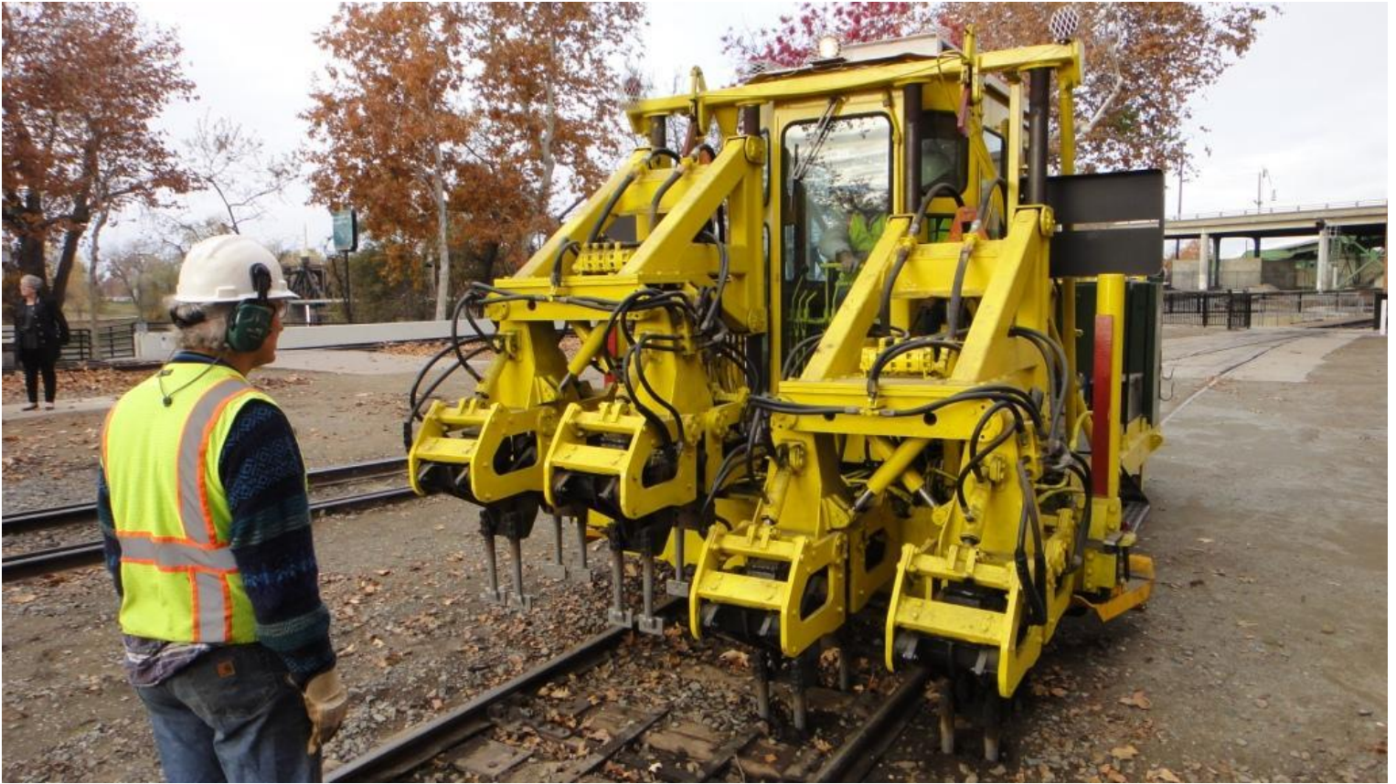
Steve N. guides the tamper around all the switch components
