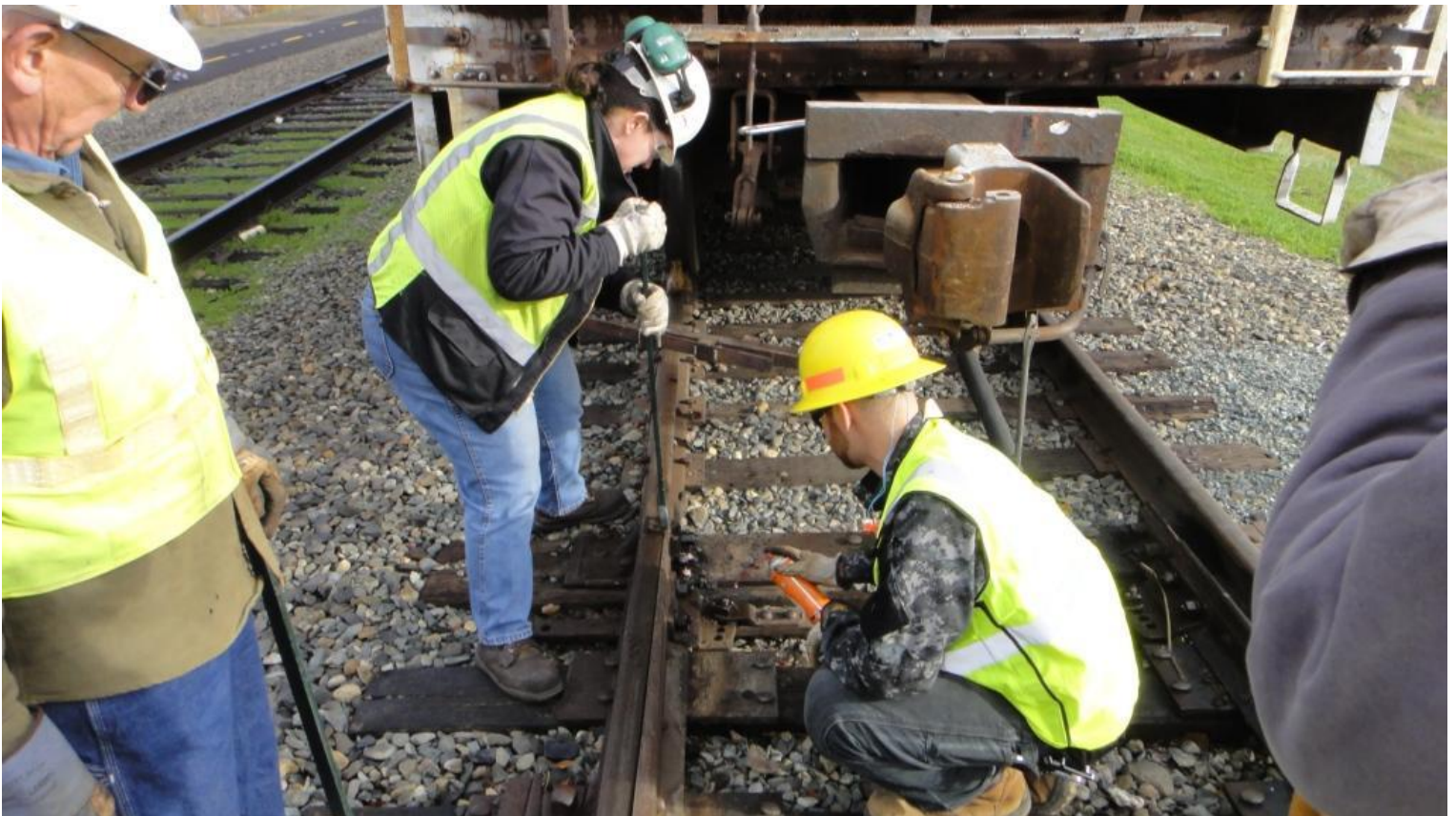
Heather and Chris remove the extraneous component from the switch point (with a little squirt of Kroil to loosen things up)
