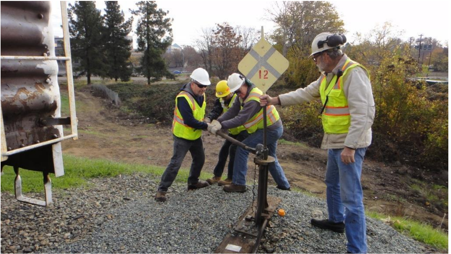
Alan guides Steve W., Chris, and Steve N. as they twist the switch stand into a new shape
