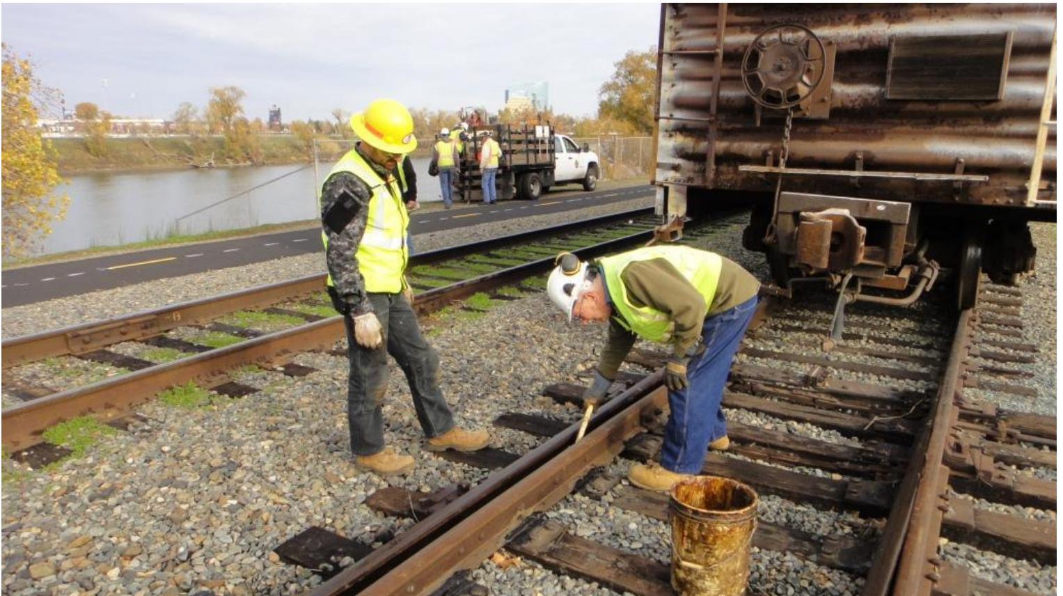
Chris watches as Clem greases the switch plates
