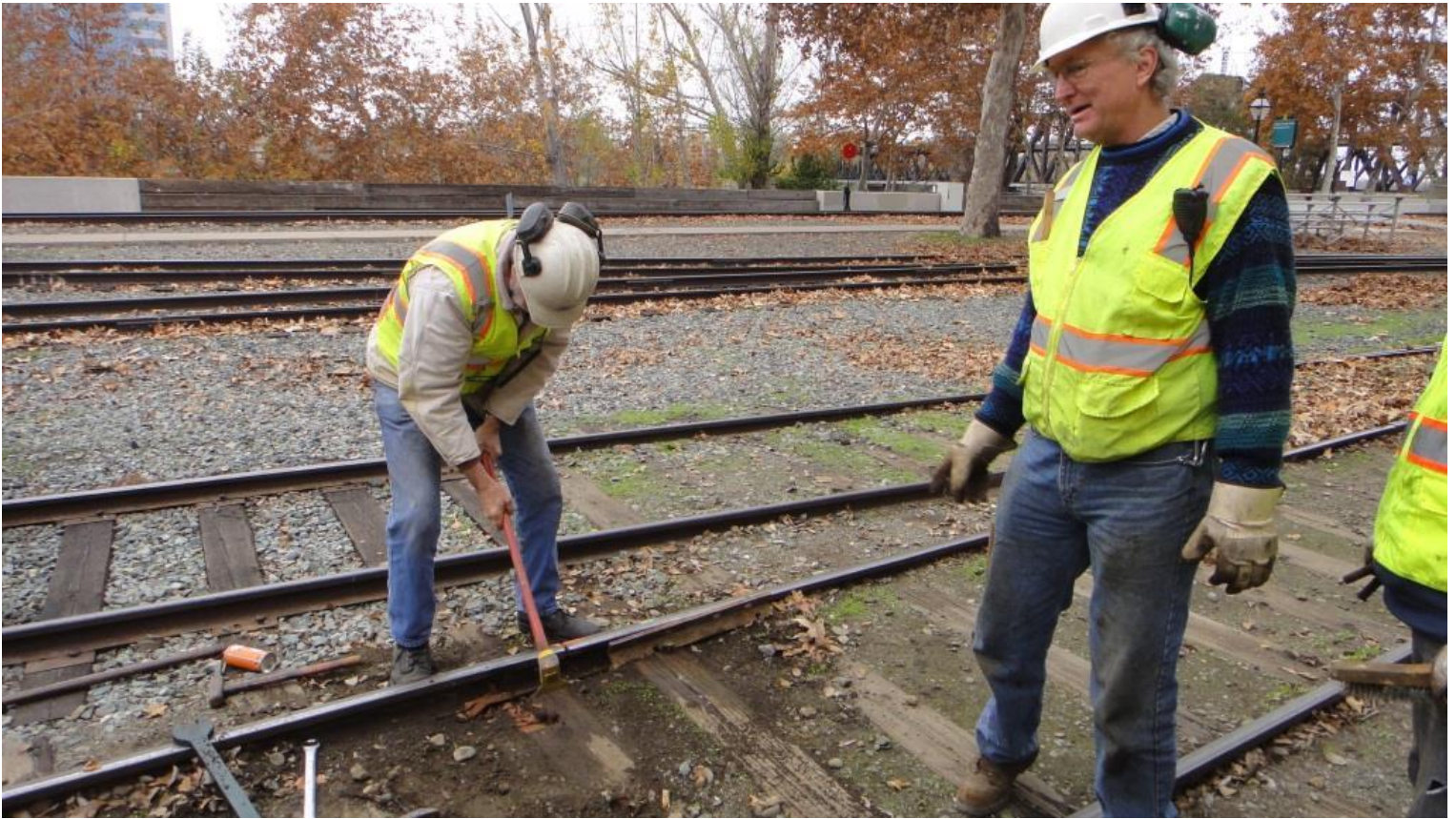
Alan uses his favorite tool, the adz, to chip-away at the tie where the base of the rail has cut into it over the years
