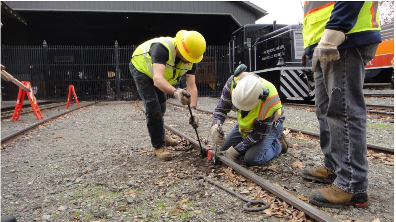
Chris and Steve N. work in tandem to remove bolts around a cracked joint-bar
