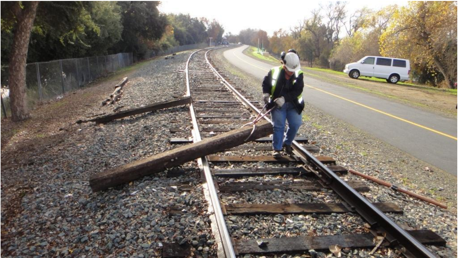
Heather spots a tie for disposal
